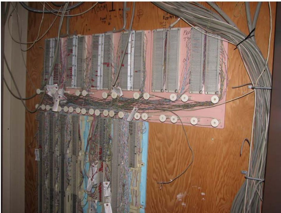
A typical closet-sized IDF.
