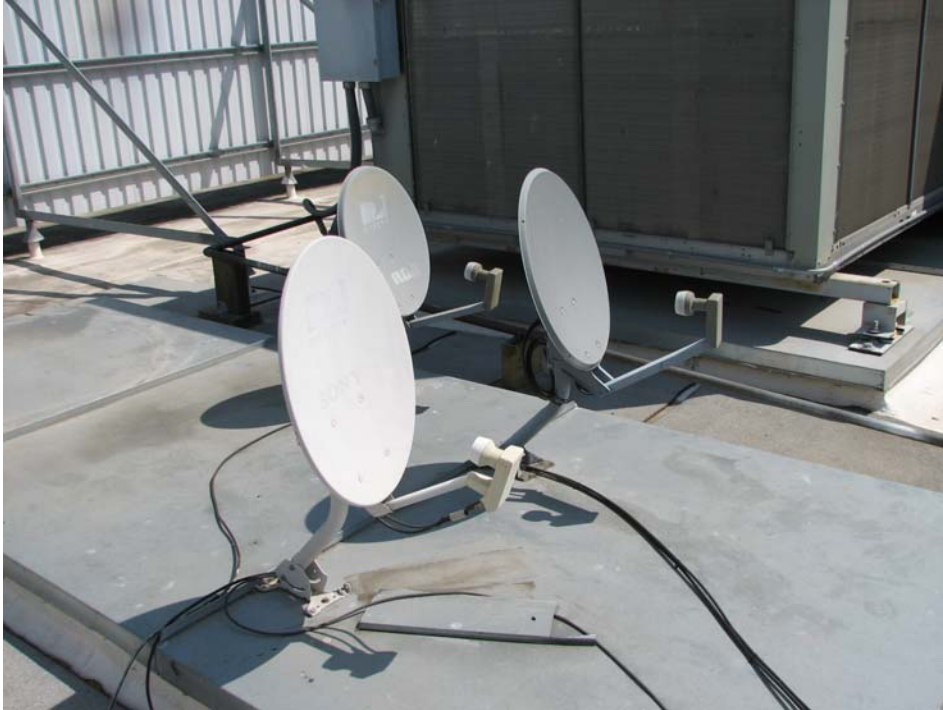
Satellite dishes located on the roof of Building 2465.
